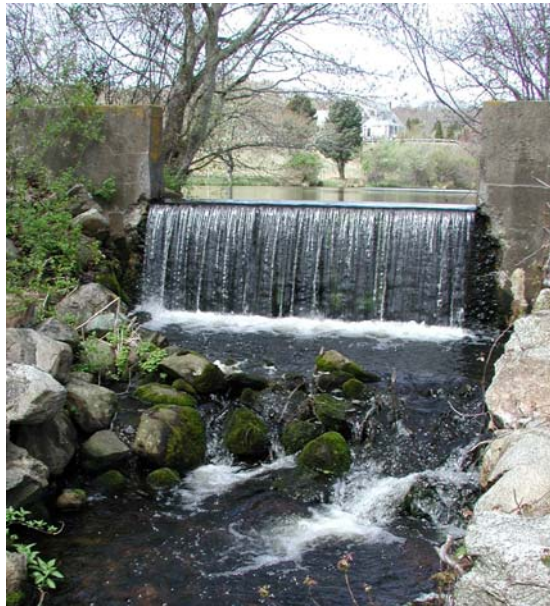
Looks Pond Dam
