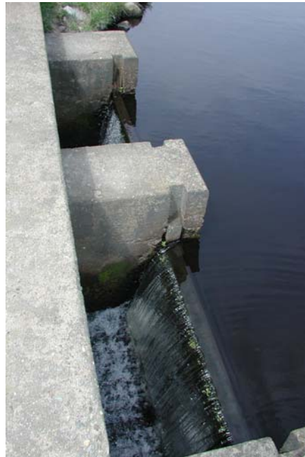
Spillway at Old Millpond Dam
